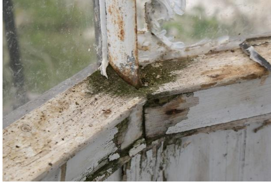
The windows are cracked and leak and the tower platform is sagging.
