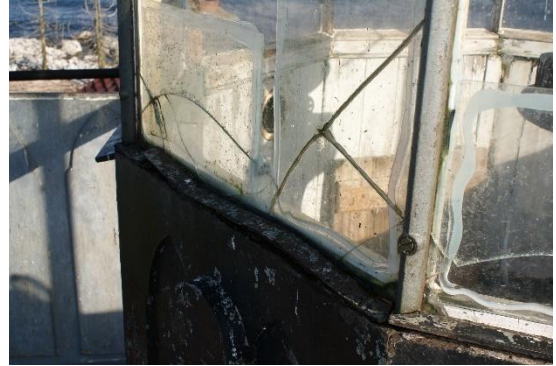
The windows are cracked and leak and the tower platform is sagging.
